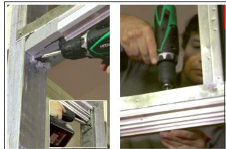
Multiple anchor points for a firm fixation
