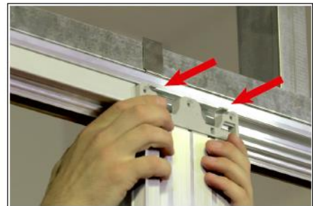
Vertical profile easy insertion by a simple "click"
