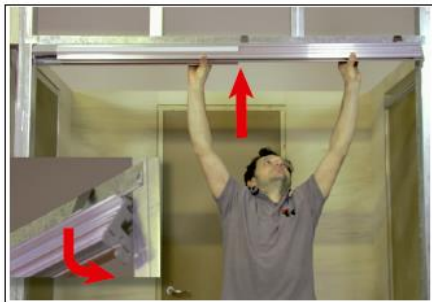
Easy Aluminum beam clipping
