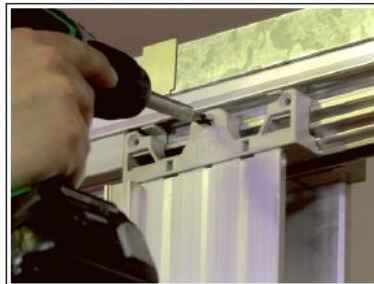
The vertical profile & the aluminum beam fixed together by screwing create a unique pocket door structure
